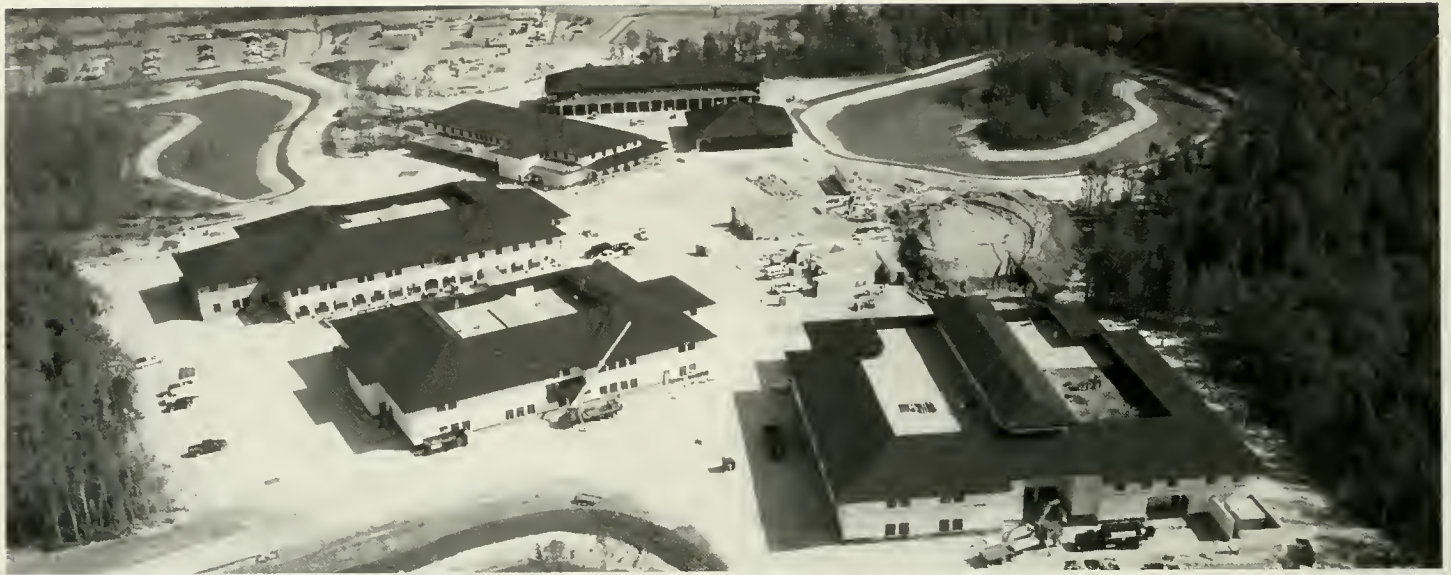
Phase One includes a nine-building complex totaling 250,000 gross sf, on a 760-acre site that is almost half jurisdictional wetlands. Photograph: Florida Aerial Services
